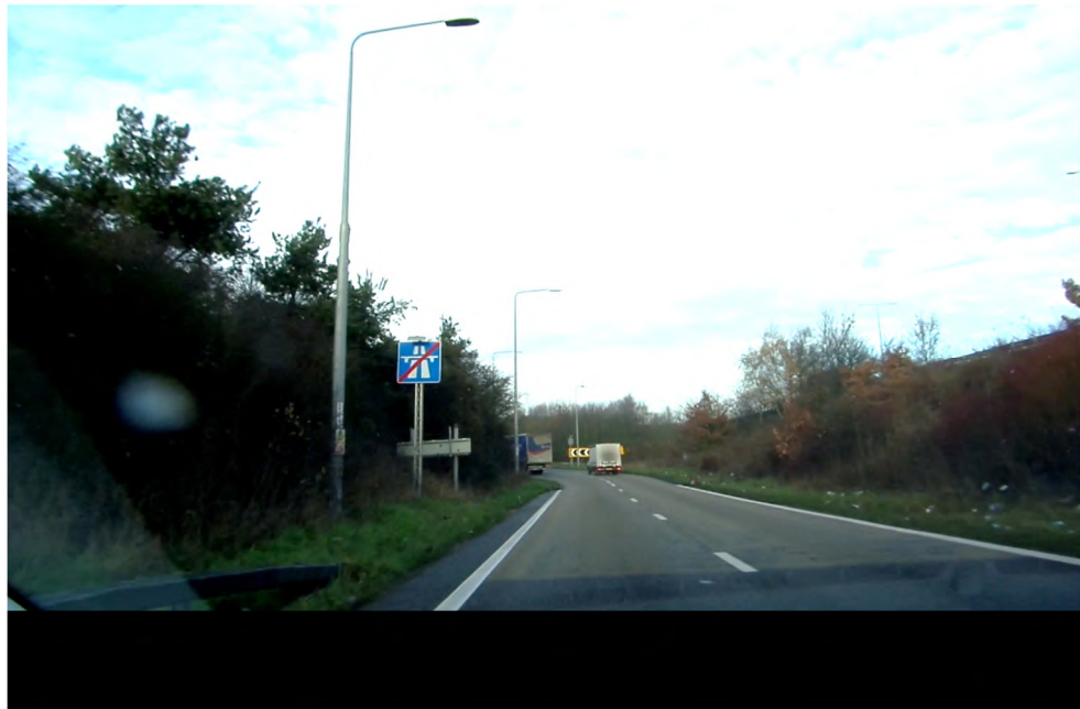
Figure 2-1 M25 northbound off-slip towards the roundabout
